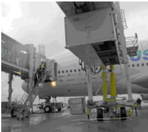
Figure 2. Ground power unit connected to an aircraft at the gate.
